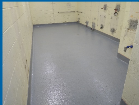
Installation of Epoxy Floor in Restrooms at Building 2020 and 2021
